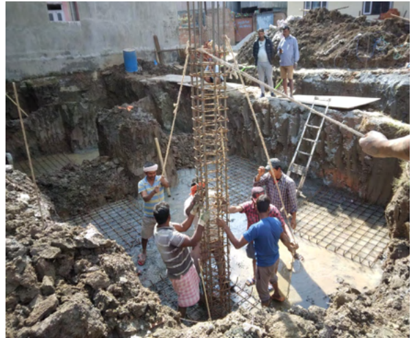
Building Foundation Work
